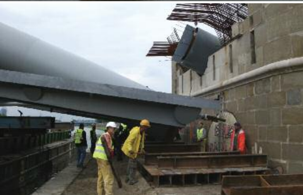
FOOTBRIDGE, KRAKOW, POLAND
