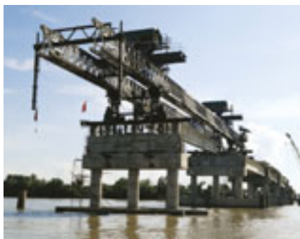
3 Each span consists of six 40m T-girders, each weighing 120t.
