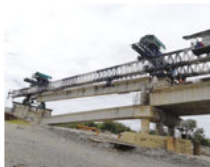
4 The most challenging part for the team was the 6.5% gradient for launching the first span on each side.
