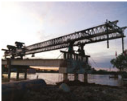
1 The River Rimbas Bridge is a simply supported bridge located in Pusa Town, Sarawak, Malaysia.
