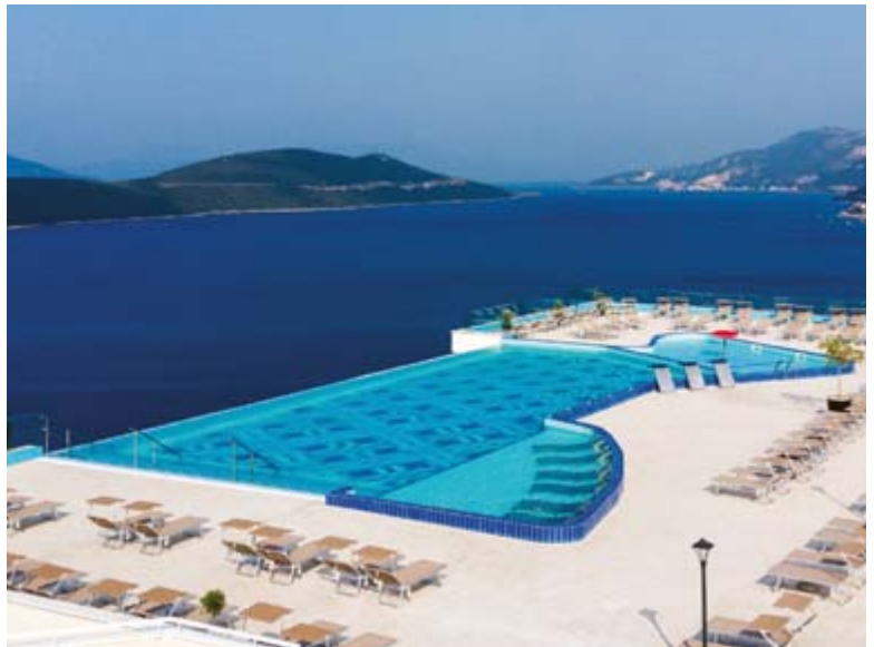
Extension work at the Grand Hotel Neum featured three floors of post-tensioned concrete slabs which have created basement level hotel delivery space, a ground floor conference suite and a 1.6m deep swimming pool & terrace on the rooftop.
