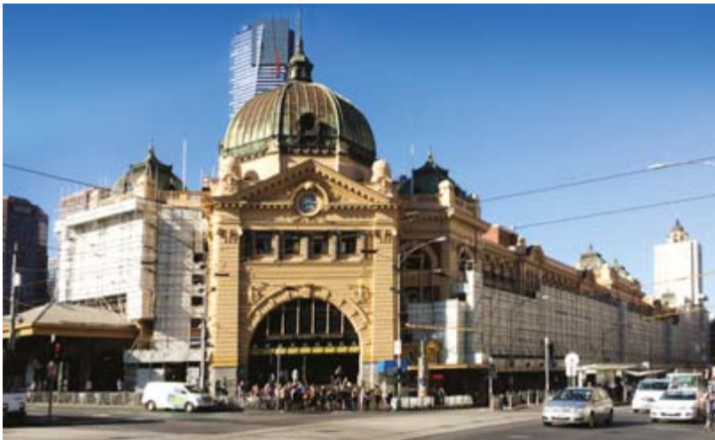
Restoration and strengthening work underway at Flinders Street Station, Melbourne.
