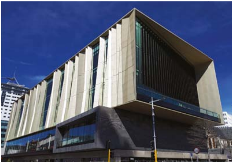
Christchurch re-imagines the library concept and the building is now restored and strengthened with the help of BBR Contech.
